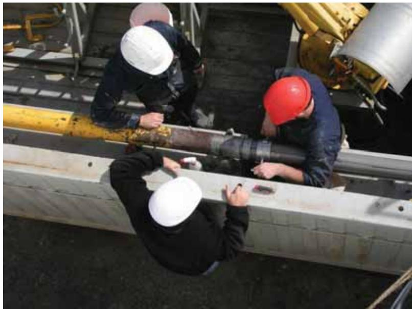
Figure 6.3 Cutting a 10 ft liner section in the half height container.
